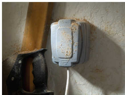
Dust proof connection to safeguard work areas.
